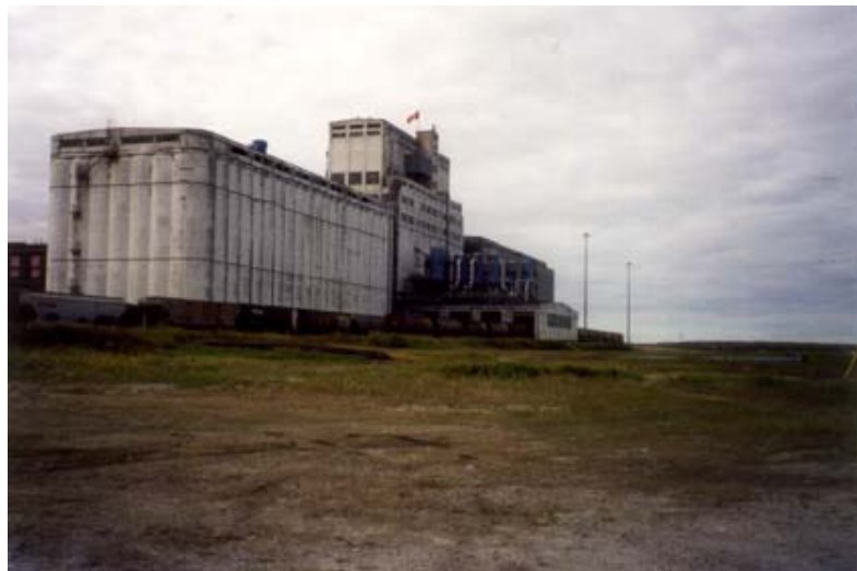
Grain elevator located just outside of Churchill.
